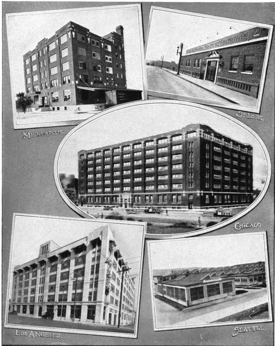
On this page and the one following are shown some of the new Westinghouse Electric Combination Sales, Service and Warehouse Buildings
